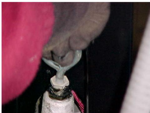
11. Open bleed valve (threaded handle)
